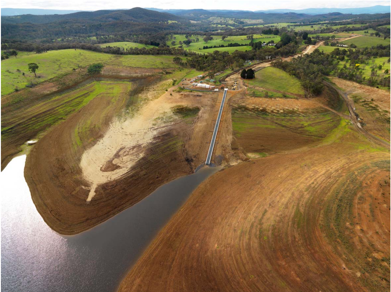
Sugarloaf Reservoir chute
