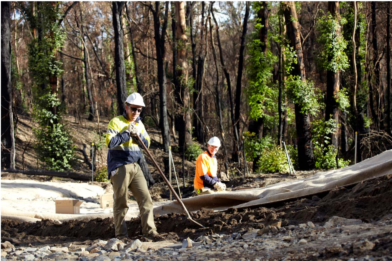
Alliance workers reinstate a creek on the Sugarloaf Pipeline alignment
